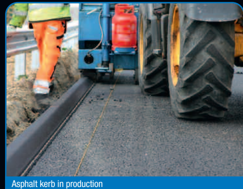
Asphalt kerb in production
