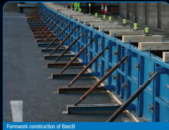
Formwork construction of BsecB
