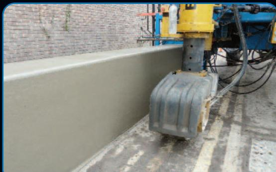
Slipform construction of BsecB
