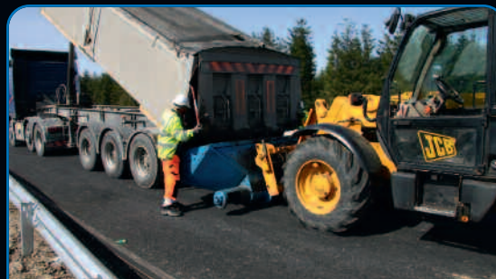
Asphalt material delivery
