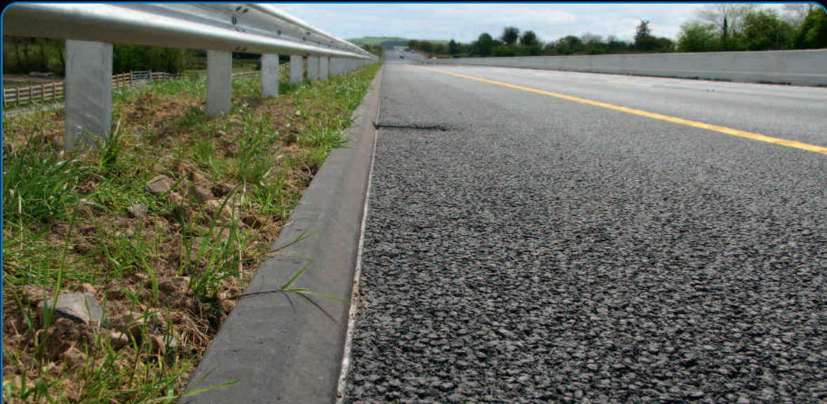
The new M7 / M8 Portlaoise to Castletown and Cullahill Motorway
