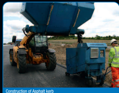
Construction of Asphalt kerb
