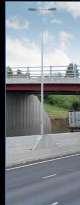
*Twin barrier accommodating level difference in excess of 300mm with localised light column plinths*
