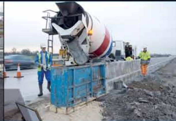
We have designed and fabricated a number of variable profile moulds including standard and wide troughed Concrete Step Barrier and support this technology with meticulous planning and clear, decisive communication with our project partners.
