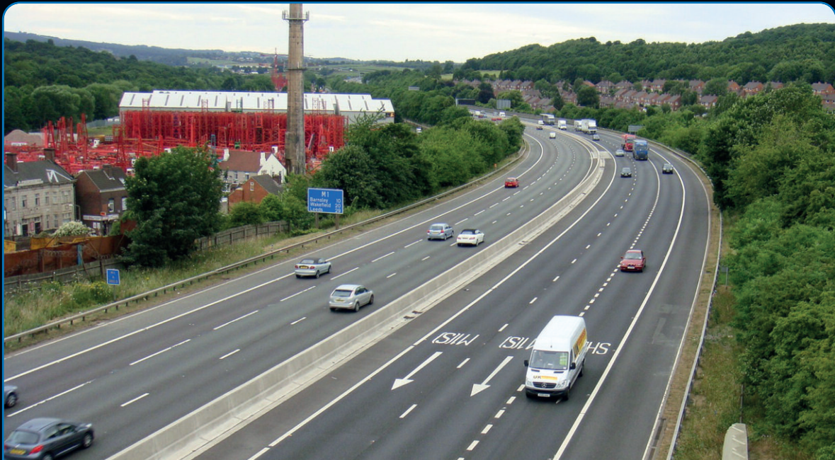
Concrete Safety Barrier on the M1 between Junctions 34 and 35
