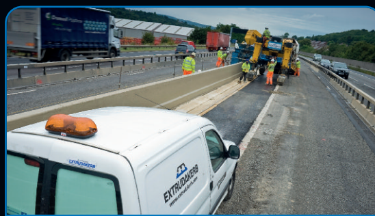
Concrete Safety Barrier under construction
