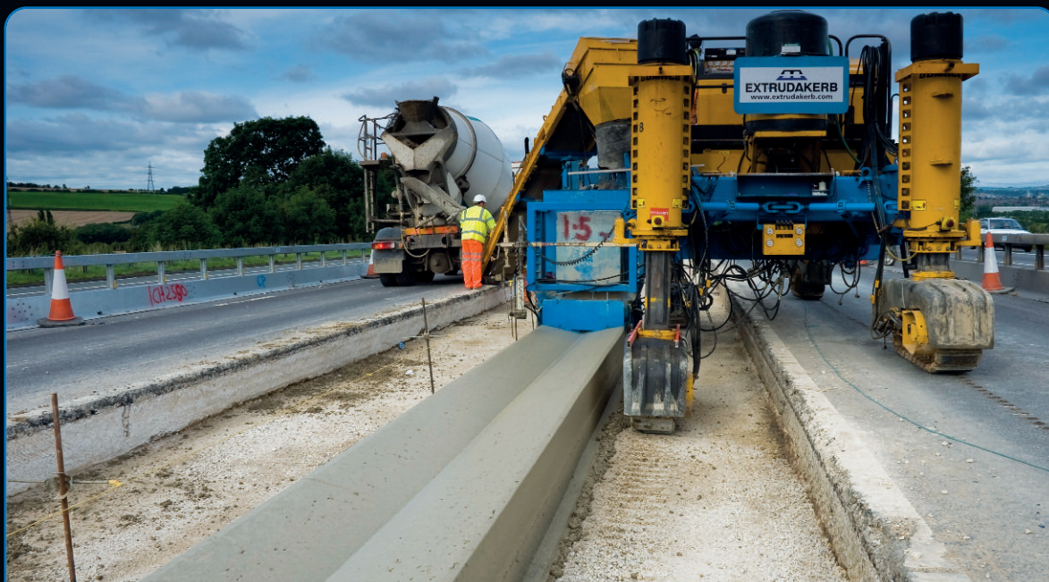
Surface Water Drainage Channel under construction
